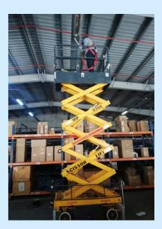
ACT installed 80W new lighting units at overhaul workshop instead of all the old traditional High Bay 250W Sodium lighting units. While in the operation and admin buildings, all the old lighting units were replaced by a new higher illumination, better intensity and energy saving 48W LED lighting units.
