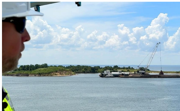
The deepening of the harbor to 50 feet began in 2021. Alabama held a ribbon cutting celebration to mark project completion in October 2025
