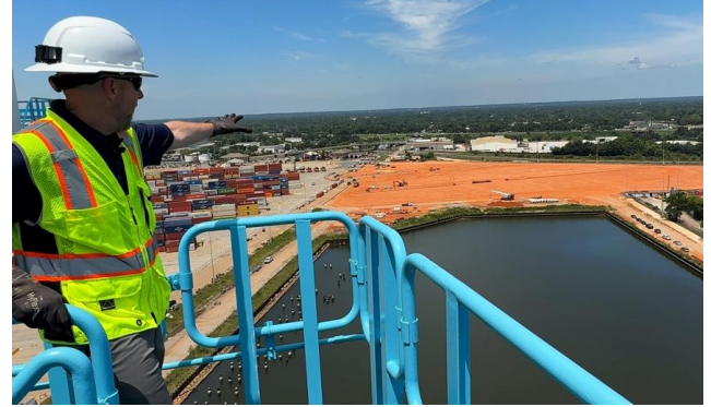
APM Terminals Mobile Managing Director Brian Harold surveys the Phase IV terminal expansion site from atop of the terminal's new super post-Panamax cranes.
