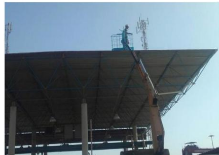
Rooftop repair – Aqaba
