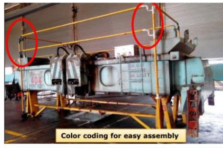
Spreader maintenance platform - GTI
