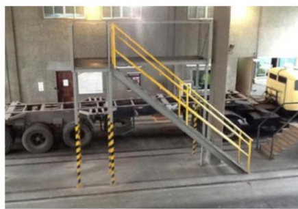
Gate inspections - External
