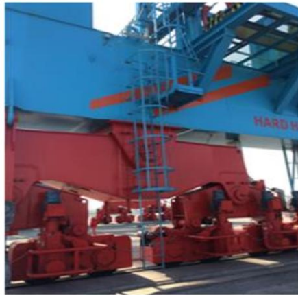
Vertical Ladder safety hoop / monkey cage
